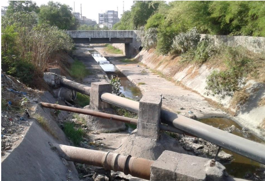
Figure 2-3: Open storm water drain in Vapi, Gujerat (Photo Vössing)
