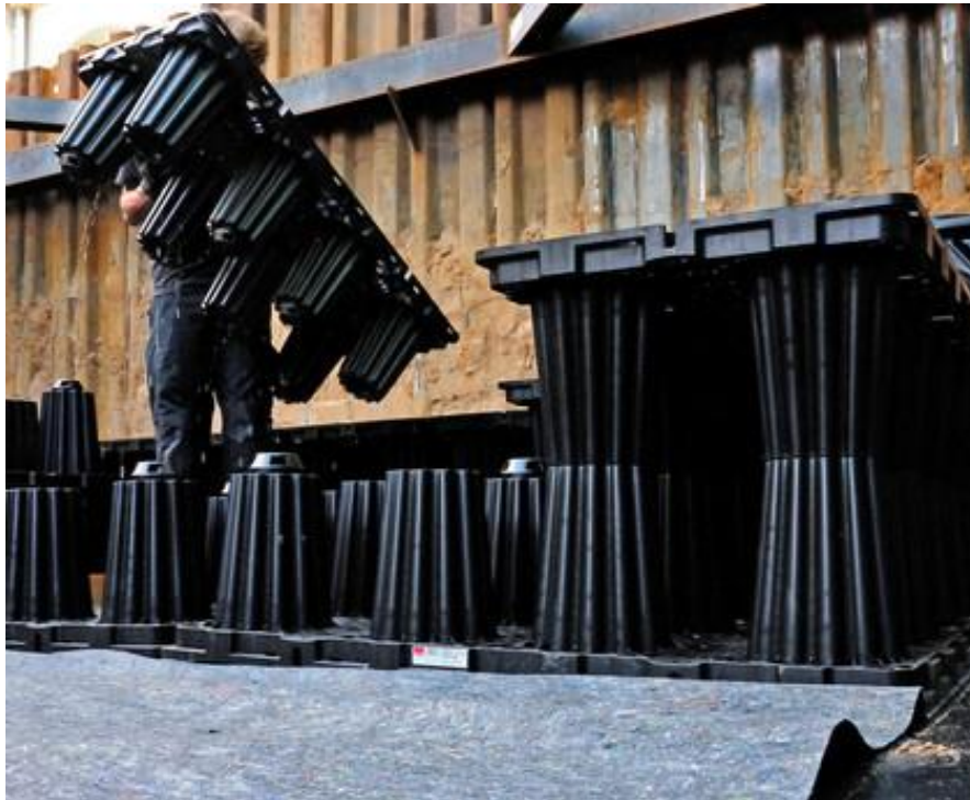
Figure 2-14: Example for hollow body elements for storm water storage "Stormbricks" (Photo:ACO)
